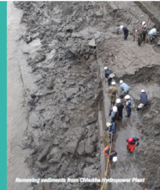
Removing sediments from Chhukha Hydropower Plant
